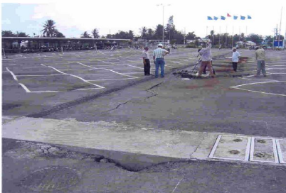
Fig. 14. Differential settlement of Hung Loi Metro project
